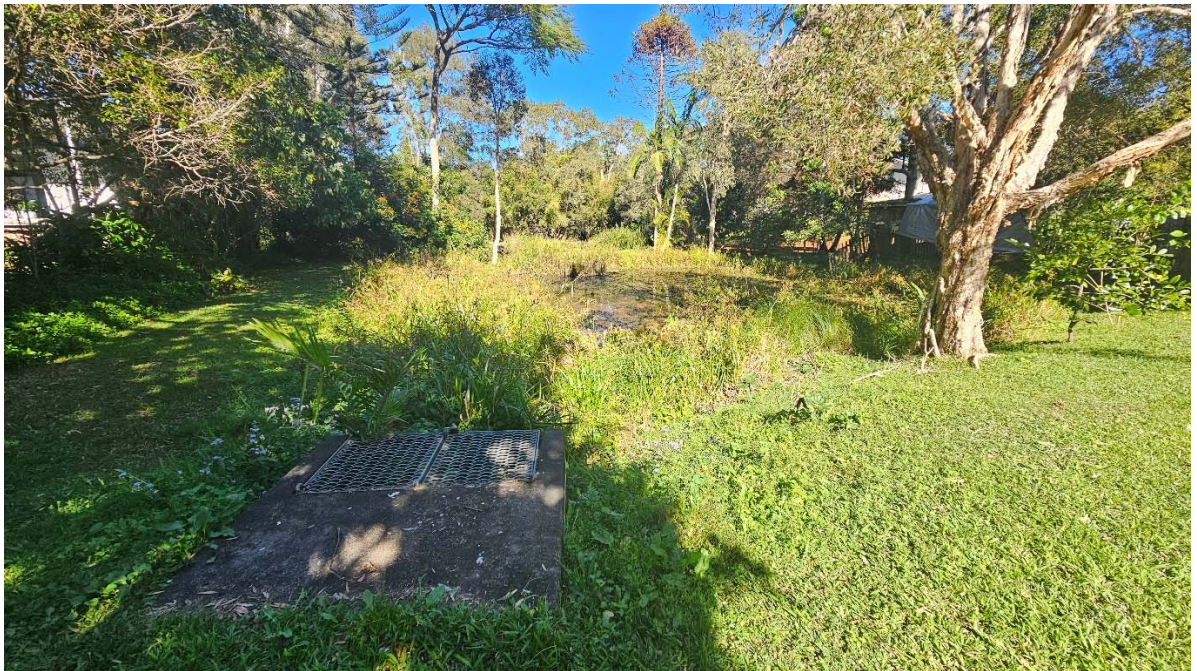
Image 4 – 900 dia outlet into existing western basin on Lot 1 DP 1007401
