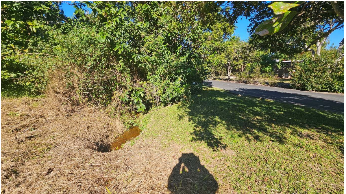
Image 3 –Eastern catchment inlet headwall
