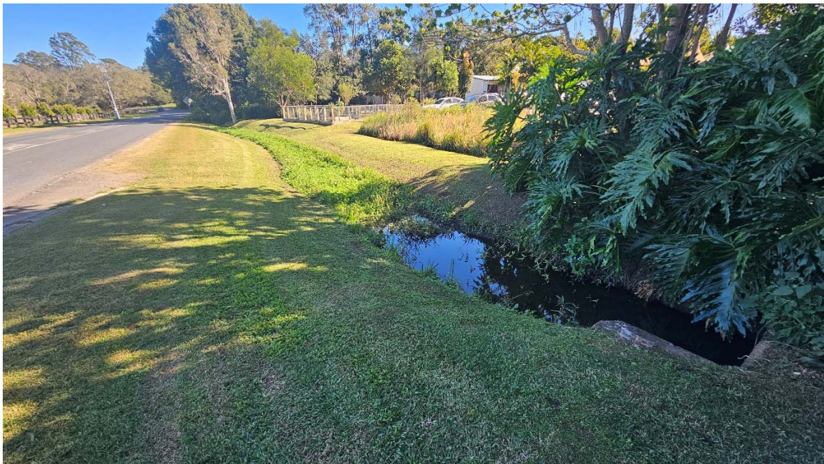
Image 6 - Left Bank Road swale
