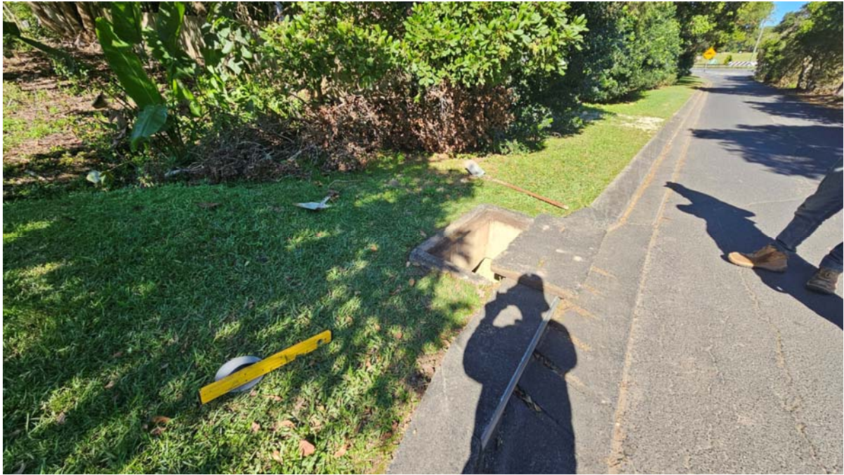
Photo 2 – Tuckerroo Ave – Kerb inlet pit with 675 outlet
